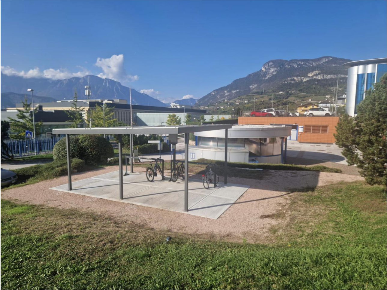
Figure 8: Photovoltaic canopy with bicycle parking at the via Sommarive site
