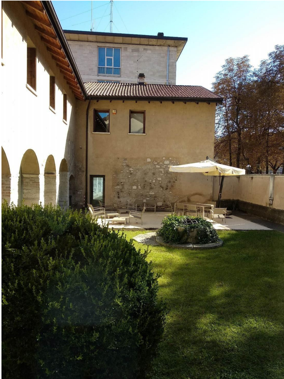
Figure 3 the Foundation's hub located on via s. Croce 77, Trento
